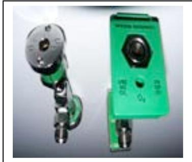
Photo #1 - Ohio and Chemtron oxygen Quick Disconnects
